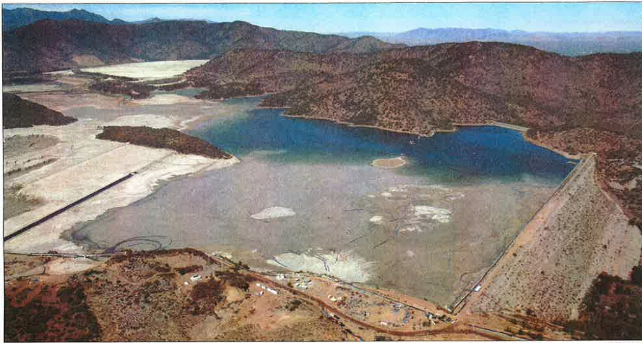
The Colihues tailings pond holds waste from Codelco's El Teniente copper mine near Rancagua, Chile. Amerigo Resources extracts copper and molybdenum from the tailings at its nearby MVC plant.
